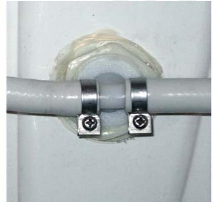
*Stainless steel pipe clips as used on Di Vapor Steam Showers.*
