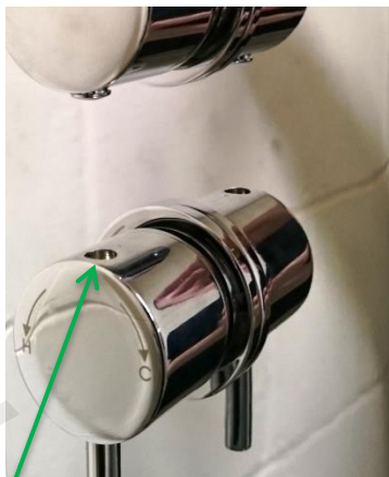
1. Remove the Temperature Handle concealing cap.
