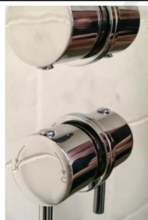
9. Re-fit the Temperature Handle Concealing cap.
